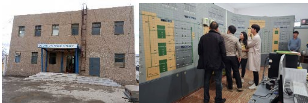
Figure 8: Project Building as Central Dispatcher Station (Source: PMC's Field Missions in October and December 2024)
