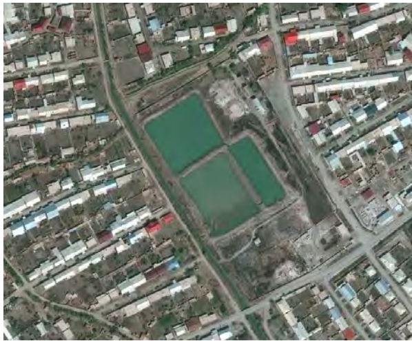
Figure 8 Current location of VU-1 Water Intake in Mangit
